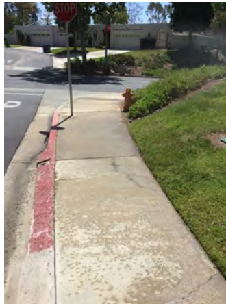
Wet sidewalk areas from overspraying sprayheads
